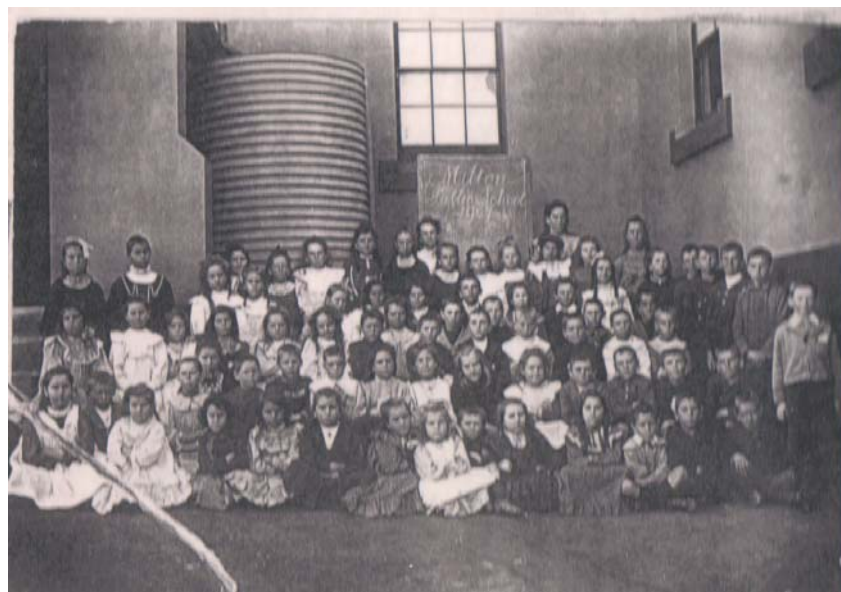
Milton Public School 1907 (noting the water tanks in the rear)
